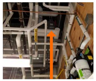
Air handling unit with no access for service, which results from of lack of site supervision during construction
