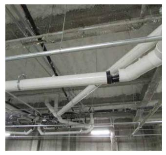
Plastic drain pipe used for beverage conduit
